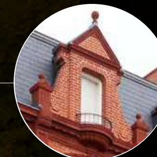
NOTABLE MANSARD ROOF
